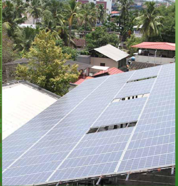
Mitsubishi Electric 25 KW Grid Solar System
